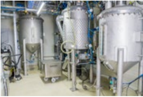
Stirrer and storage tanks for rapeseed pulping and conditioning
